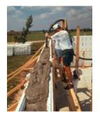
Yes. Concrete's mass increases energy efficiency because concrete walls respond to changes in temperature very slowly. For example, it may take 4 to 8 hours for a temperature change to migrate through a concrete wall,
