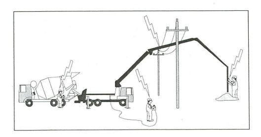
**1.3 WARNING! LIGHTNING, ELECTROCUTION HAZARD!** Although electrocution due to lightning is rare, lightning should be monitored if in the area. If you feel the risk of a lightning strike, notify the operator that you will be in the cab of the concrete delivery vehicleuntil the threat has subsided.
